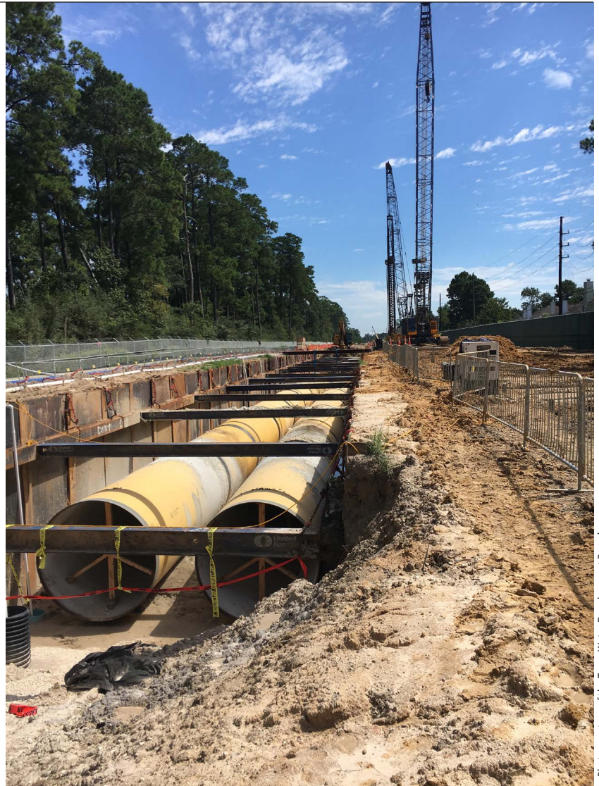
View of the Northeast Water Purification Plant expansion project in Humble
